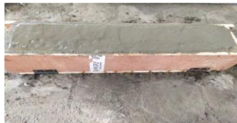
Figure 3: Casting of beam
