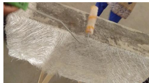
Figure 6: wrapping of beam
